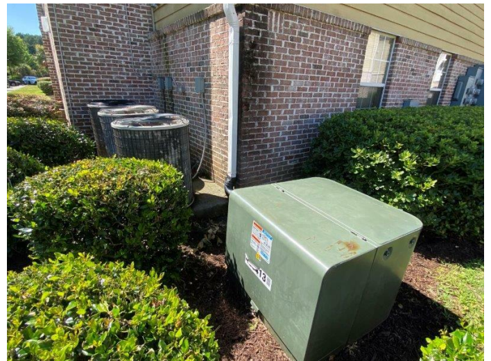
28. Representative split systems and pad-mounted transformers
